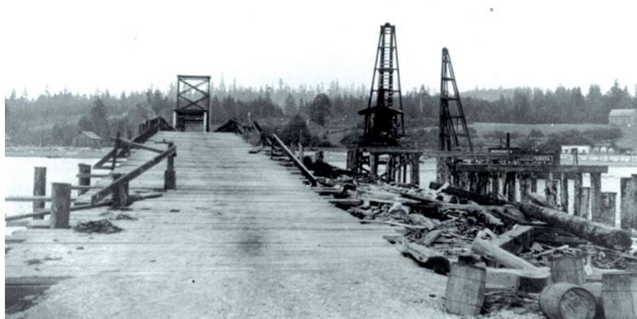
The third bridge under construction in 1920, south of the old bridge. Two pile drivers working on the new bridge can be seen on the right. This view is from Wauna looking east.
